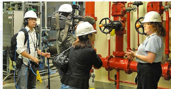
NRC Inspection Team
